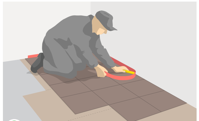
4 Perimeter insulation barrier cut
